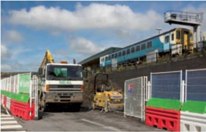
Cardiff is blessed with a city-centre rail station, served by trains on all routes. Work is under way at Cardiff Central to create an additional platform to boost capacity and reliability.
